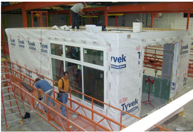
Figure 7: A home under construction in the ZETA factory www.zetacommunities.com
