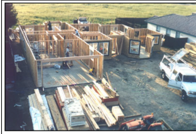
Figure 4: A pre-cut home being constructed www.caprefab.com
