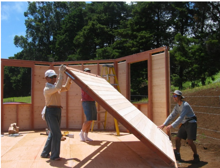
Figure 3: A panelized home being constructed www.multifacetedhomes.com
