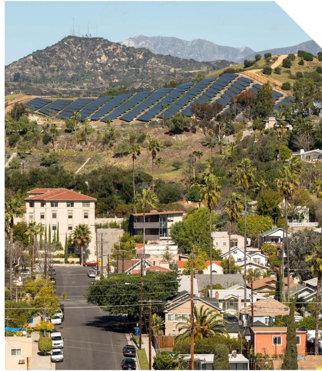
Occidental College's solar array, as seen from Highland Park.
